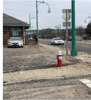
Photo 4: Partially Obstructed Sight Line (to the north)
