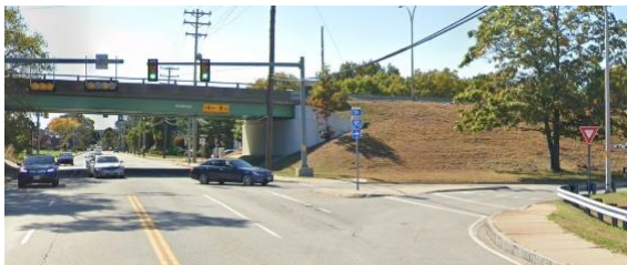
Photo 3: T.F. Green Airport Connector On-Ramp at Post Road
