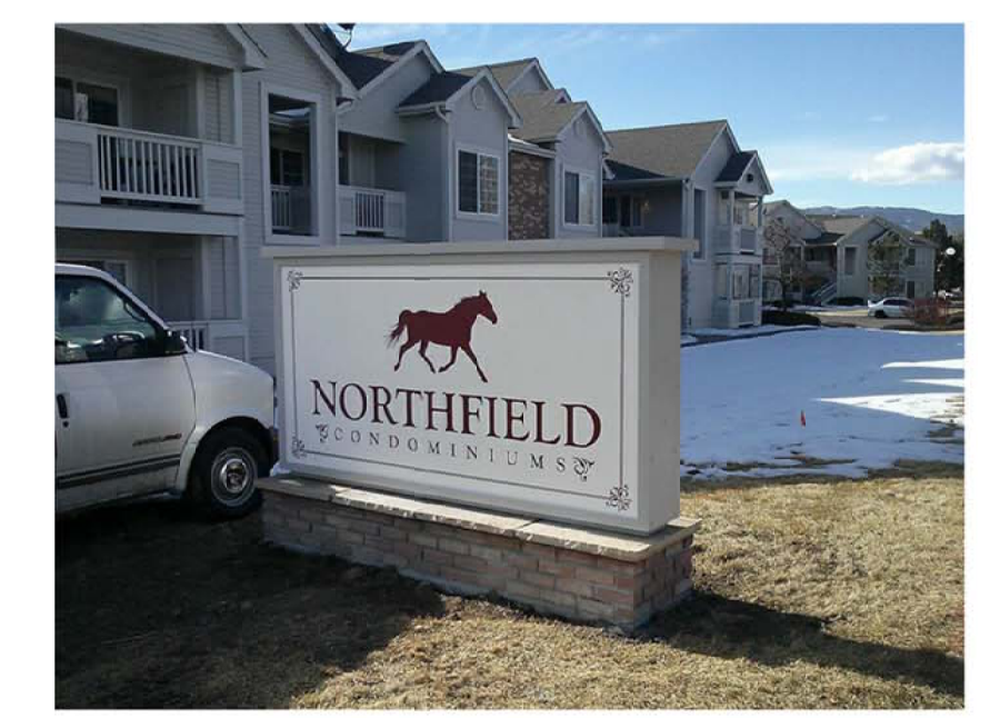
MONUMENT SIGN - CHARACTER AND STYLE PROPOSED FOR THIS PROJECT. APPROXIMATELY 2' WIDE x 10' WIDE x 4' TALL MOUNTED ON 18" STONE BASE
