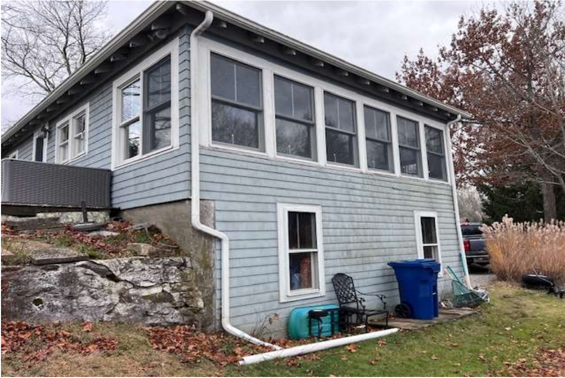
SUBJECT PROPERTY - REAR OF DWELLING
