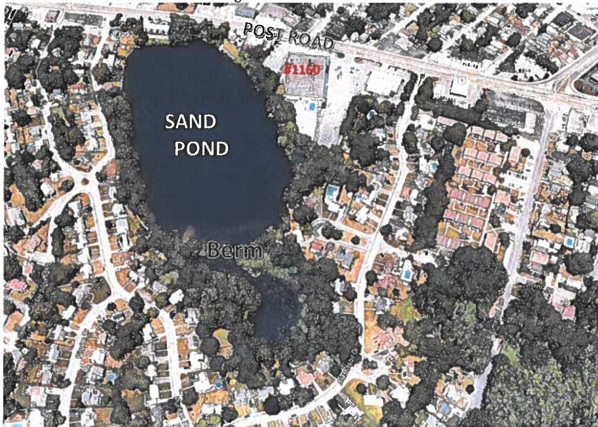
Sand Pond Aerial Photo: View Looking West towards Post Road:
