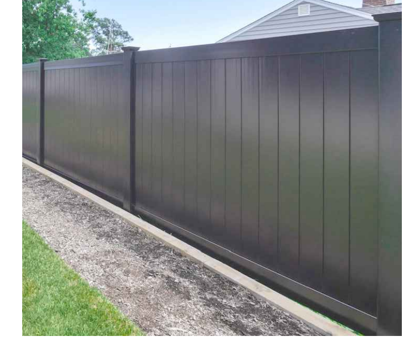
BLACK TONGUE AND GROOVE VINYL PRIVACY FENCE IMAGE SHOWN FOR ARCHITECTURAL CHARACTER OF PROPOSED PRIVACY PANELS OF ORNAMENTAL ACCESS GATE
