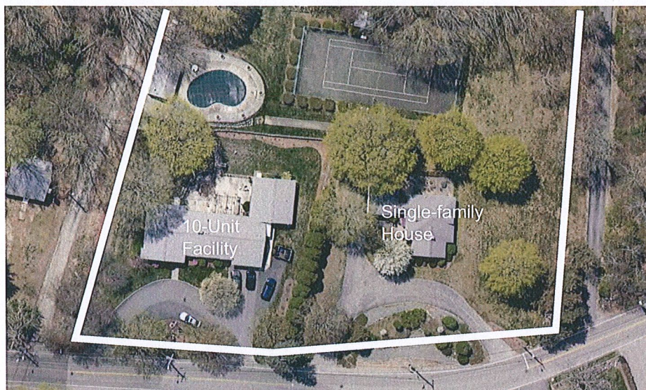
Aerial View of Site
