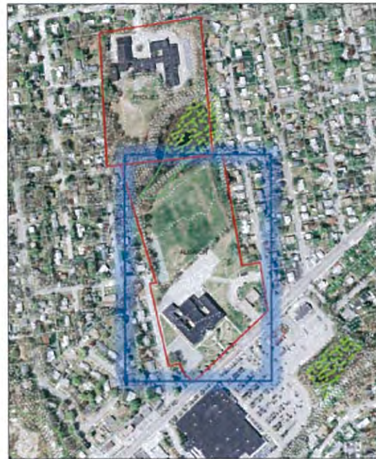
Method Type: Aerial Description: Aerial Aerial J. H. Rhodes Elementary Property (former) 789 Post Road Warwick, RI Warwick Map 145 130 800 Feet
