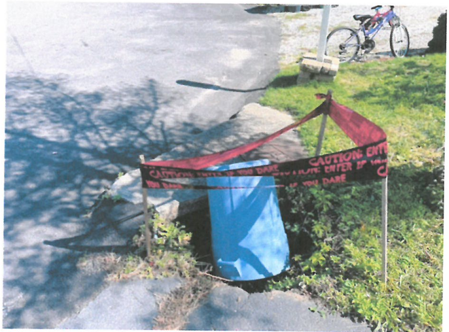
I covered the broken light pole and broken base with a trash can and put tape around hole area to help keep the neighborhood kids safe.
