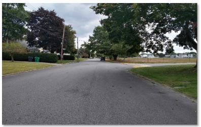
intersection. To enhance safety and enforce the yield condition operation, a raised painted crosswalk was installed across Anscot Court. This feature can be seen in the above photograph where Anscot Court yielding traffic turning onto Harmony Court must slow to manuever over the raised crosswalk positioned at the junction.
