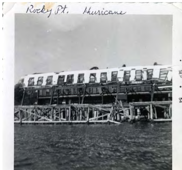
Rocky Point after Hurricane Carol, 1954 (John Greene Collection)
