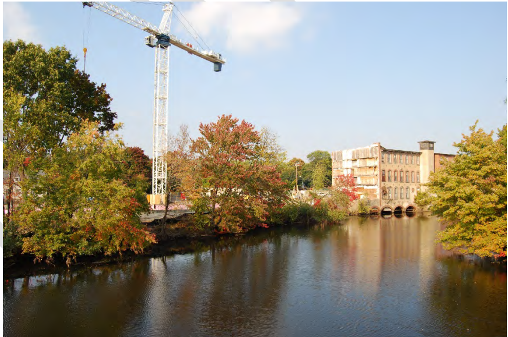
Reconstruction of Pontiac Mills (Nylo Hotel) along the Pawtuxet River after the 2010 Floods.
