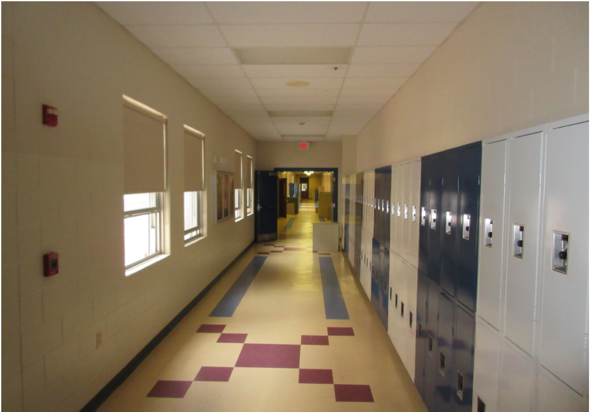
Hallway in Building Addition, Aldrich Junior High School
