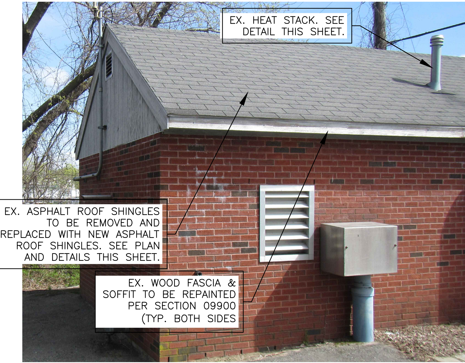
EX. STATION ROOF UPGRADES SCALE: NTS
