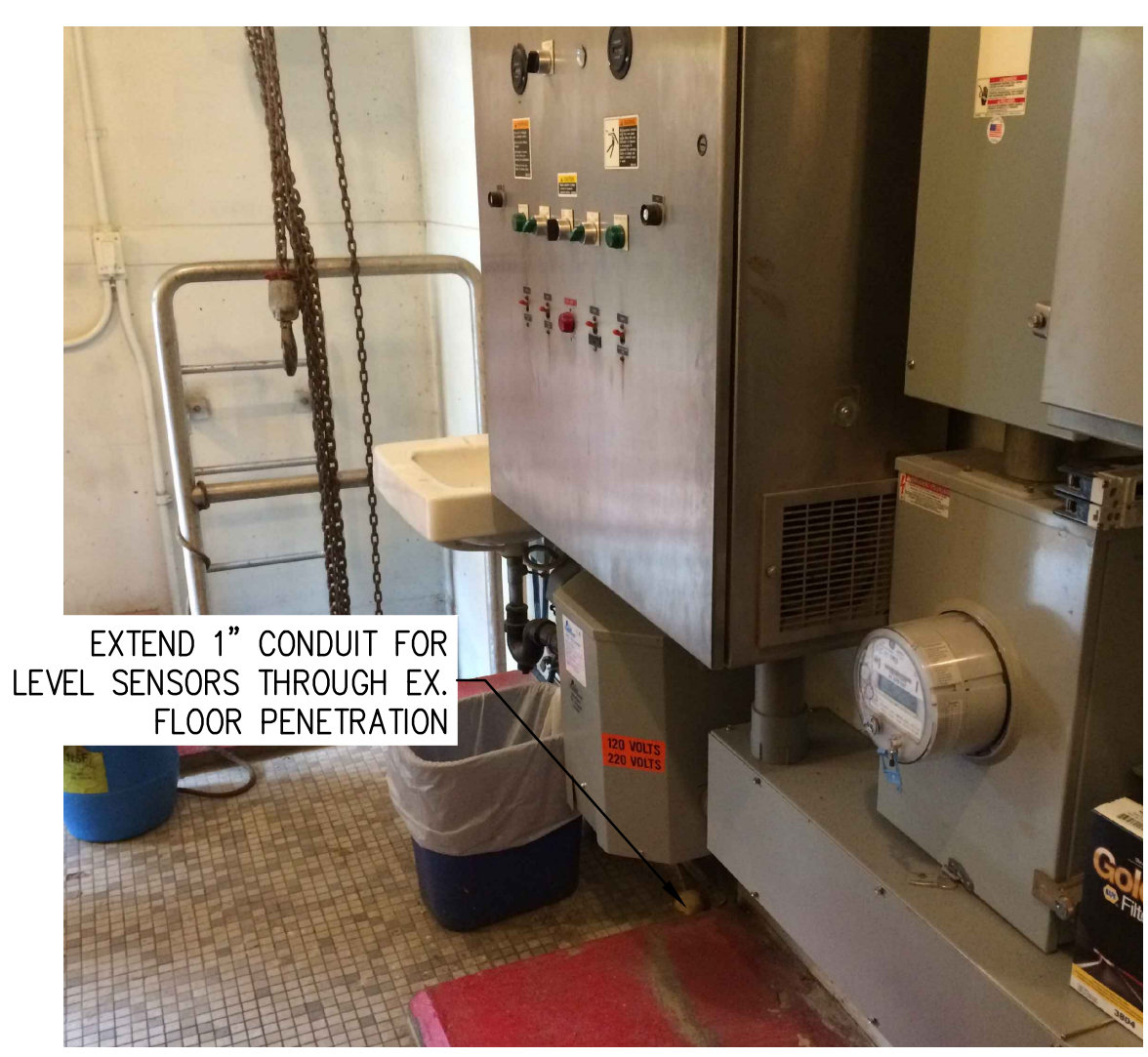
EX. WALL MOUNTED CONTROL PANEL SCALE: NTS
