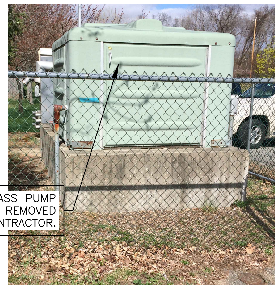
EX. FIBERGLASS PUMP SKID ENCLOSURE SCALE: NTS
