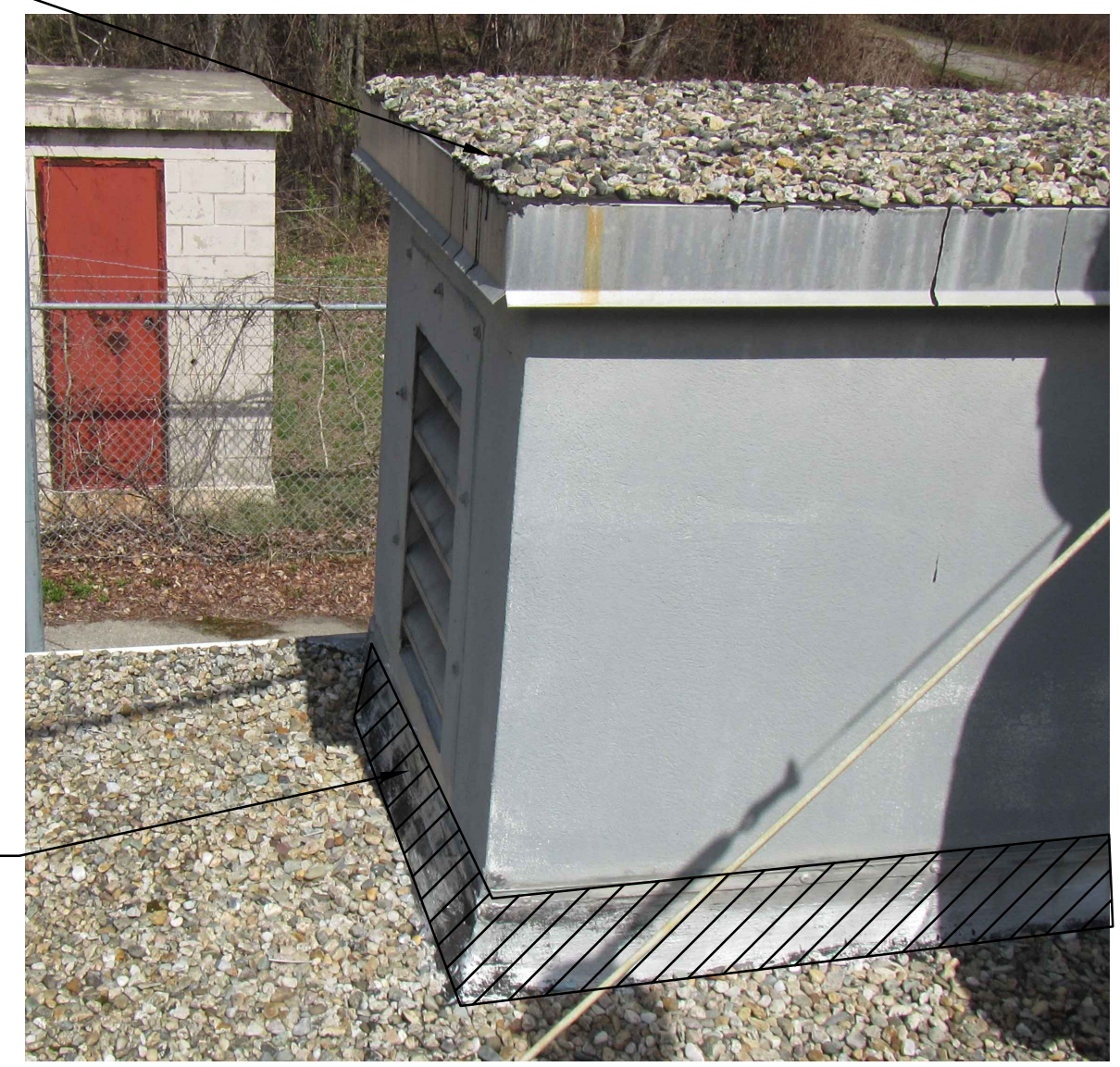
EXISTING INTAKE AIR CUPOLA - FLASHING SCALE: NTS
