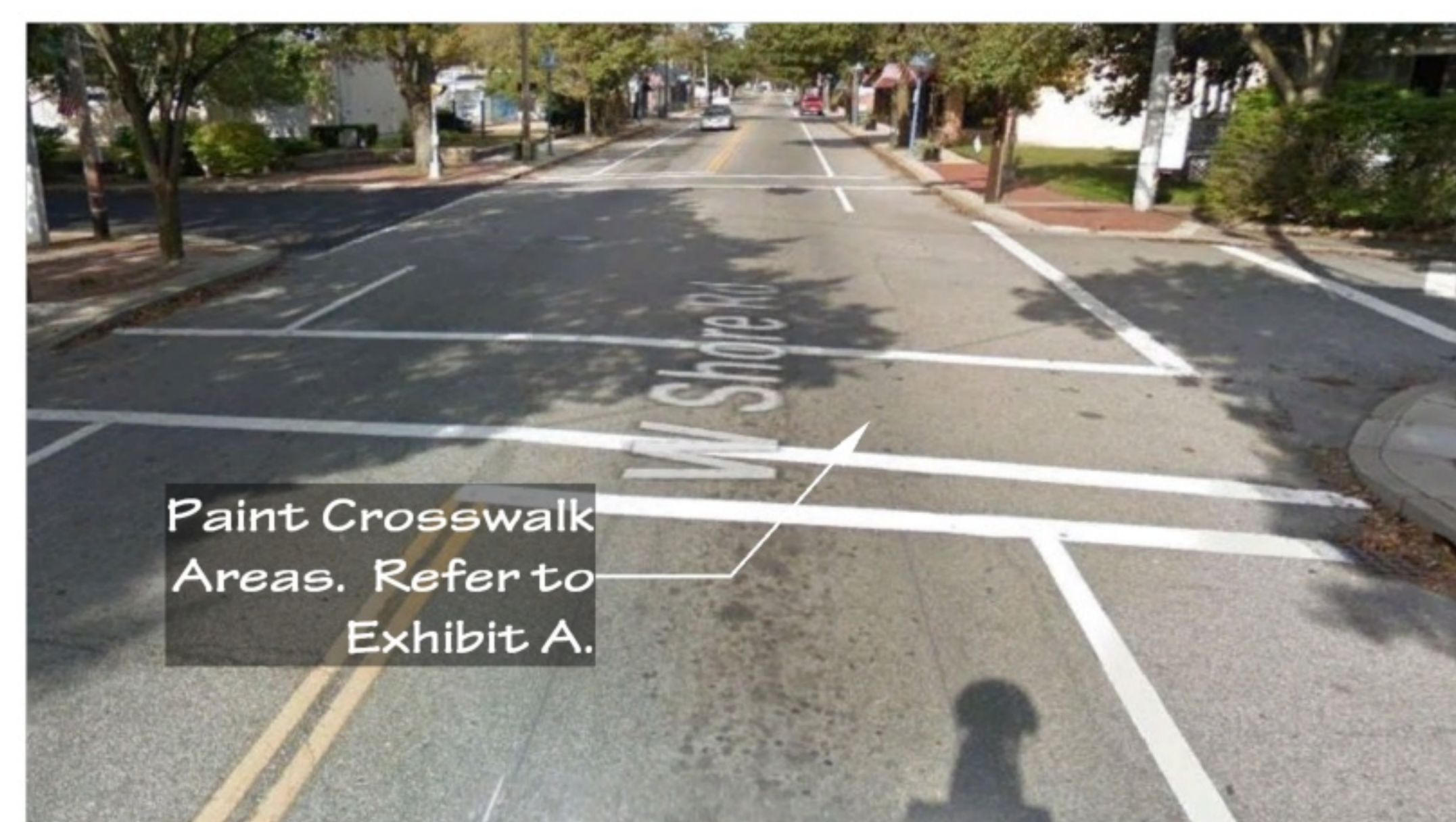
J Beach Ave./ West Shore Intersection - Paint existing crosswalks with solid brick red paint color. Contractor is responsible for all traffic control during painting operations. Refer to Exhibit A - Plans for Proposed Crosswalk Improvements, Conimicut Village Business District.
