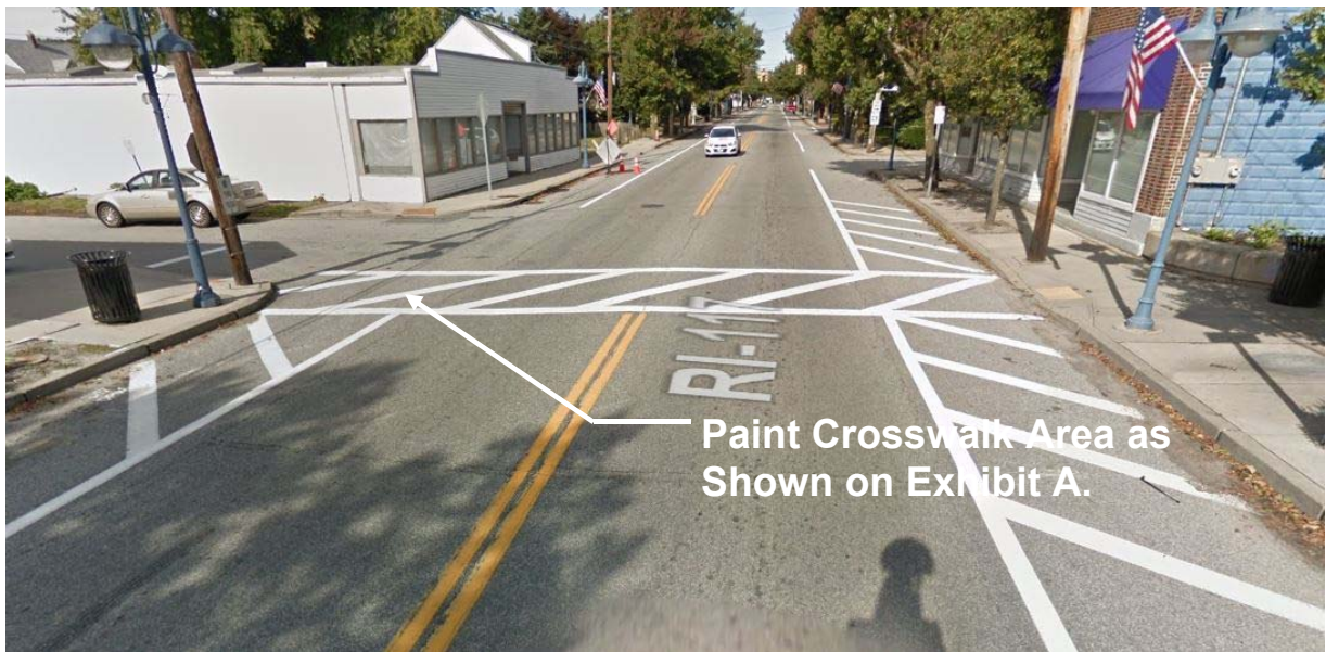
Figure 3 - Paint existing crosswalk at the intersection of Maplewood Avenue and West Shore Road as shown on Exhibit A.
