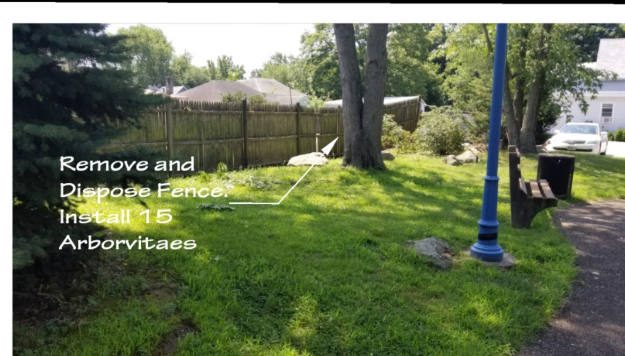
G Donovan Park - Remove and dispose of approximately 100' of existing wood fencing. Install 15 CY loam in linear 5'W X 50'L X 1.5'H berm bed and install fifteen (15) 6'-8" Emerald Arborvitae shrubs in center of berm. Install a 3" thick layer of dark pine bark mulch over entire bed area.
