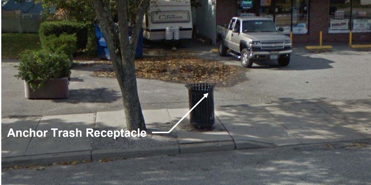
Figure 4 – Image of one of the three (3) trash receptacles that must be anchored to the existing sidewalk utilizing expansion anchors or other suitable anchoring method as approved by the Project Manager.
