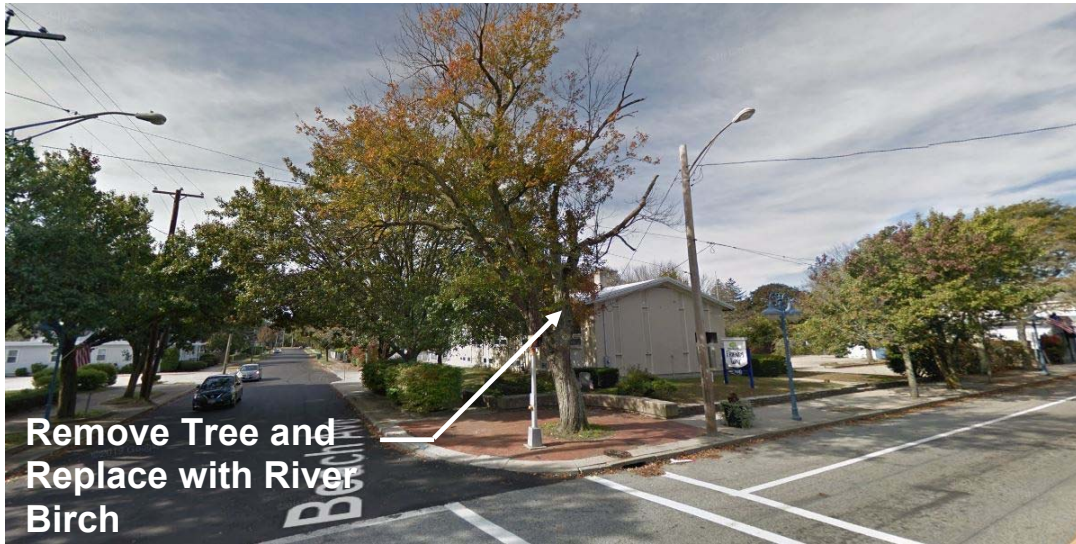
Figure 8 – Existing tree at the corner of West Shore Road and Beach Street must be completely removed. Stump must be ground to below grade and a new 12'-14' multi-stem Heritage River Birch Planted in its place. Install raised jumbo cobblestones around the edge of the circle on edge and mulch circle.
