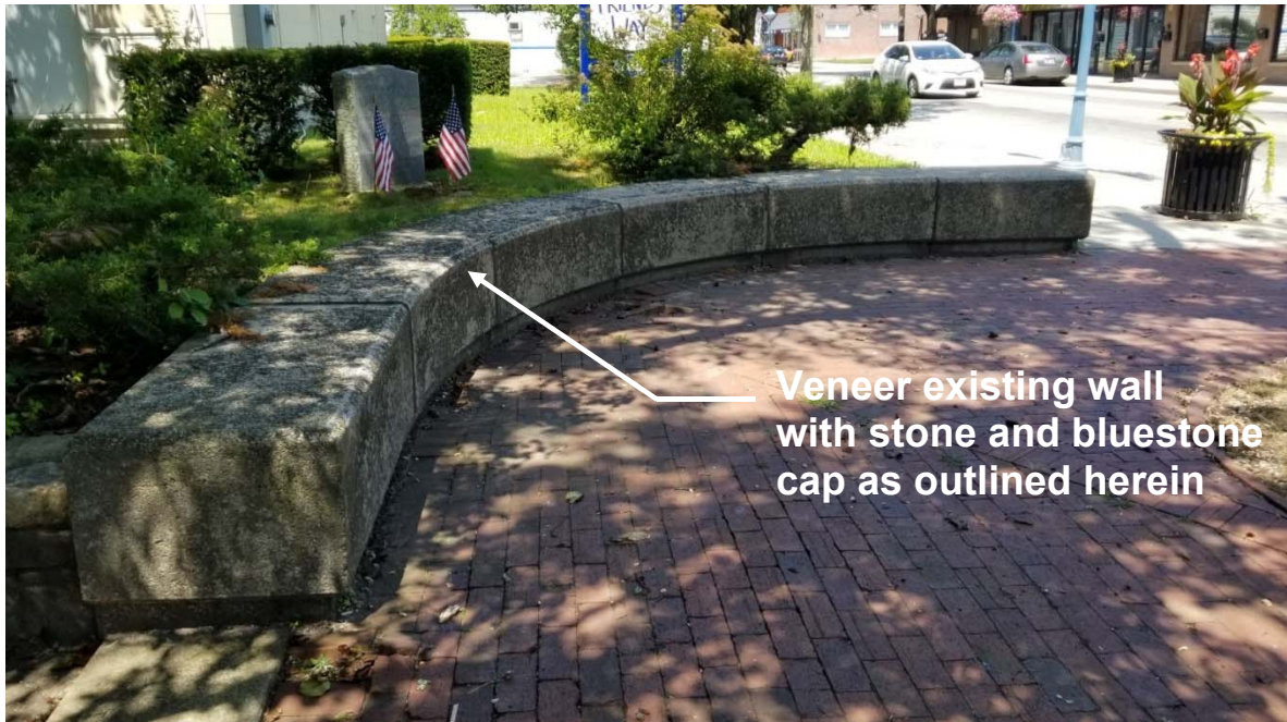
Figure 11 –Existing wall at the corner of Beach Avenue and West Shore Road. Veneer wall with natural thin stone with bluestone cap as outlined in Section 04 41 00.
