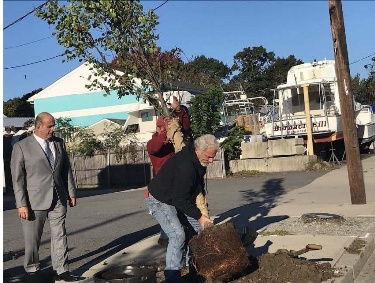
Figure 10 – Install trees in accordance with Section 32 90 00. Excavate and dispose of existing soil material, install tree, backfill with clean loam, install 3” of dark pine bark mulch, and stake tree.
