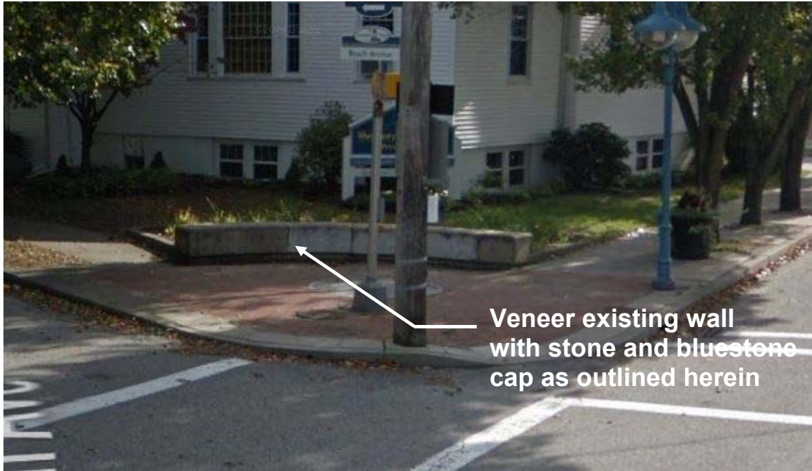
Figure 12 –Existing wall at the corner of Beach Avenue and West Shore Road. Veneer wall with natural thin stone with bluestone cap as outlined in Section 04 41 00.
