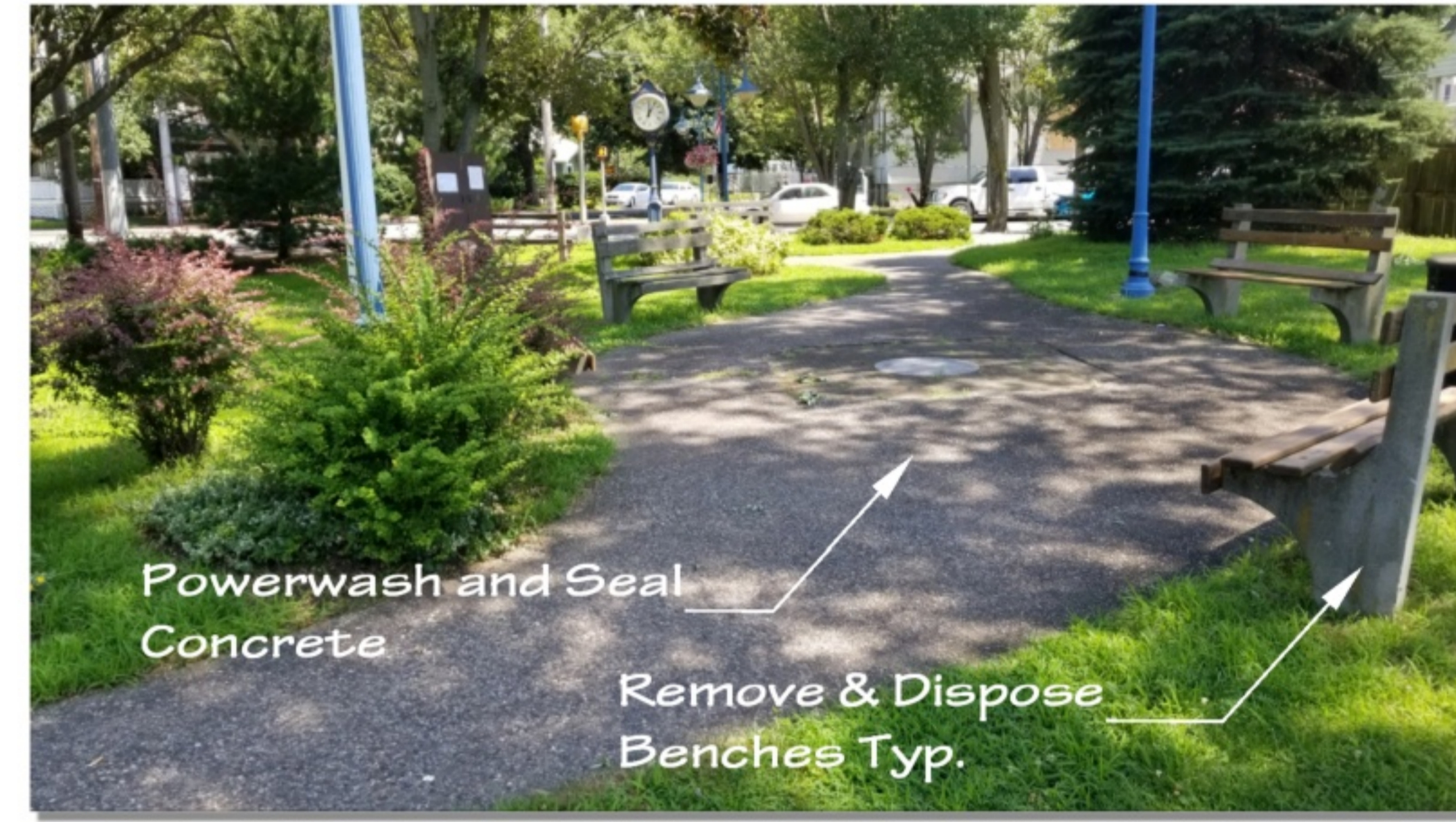
H Donovan Park - Powerwash all exposed aggregate concrete surface to remove dirt and stains. Once dry, seal concrete with Techniseal ProSeries Waterproofing Sealant for Brick and Concrete (WR7) or approved equal. Apply according to manufacturer recommendations.
