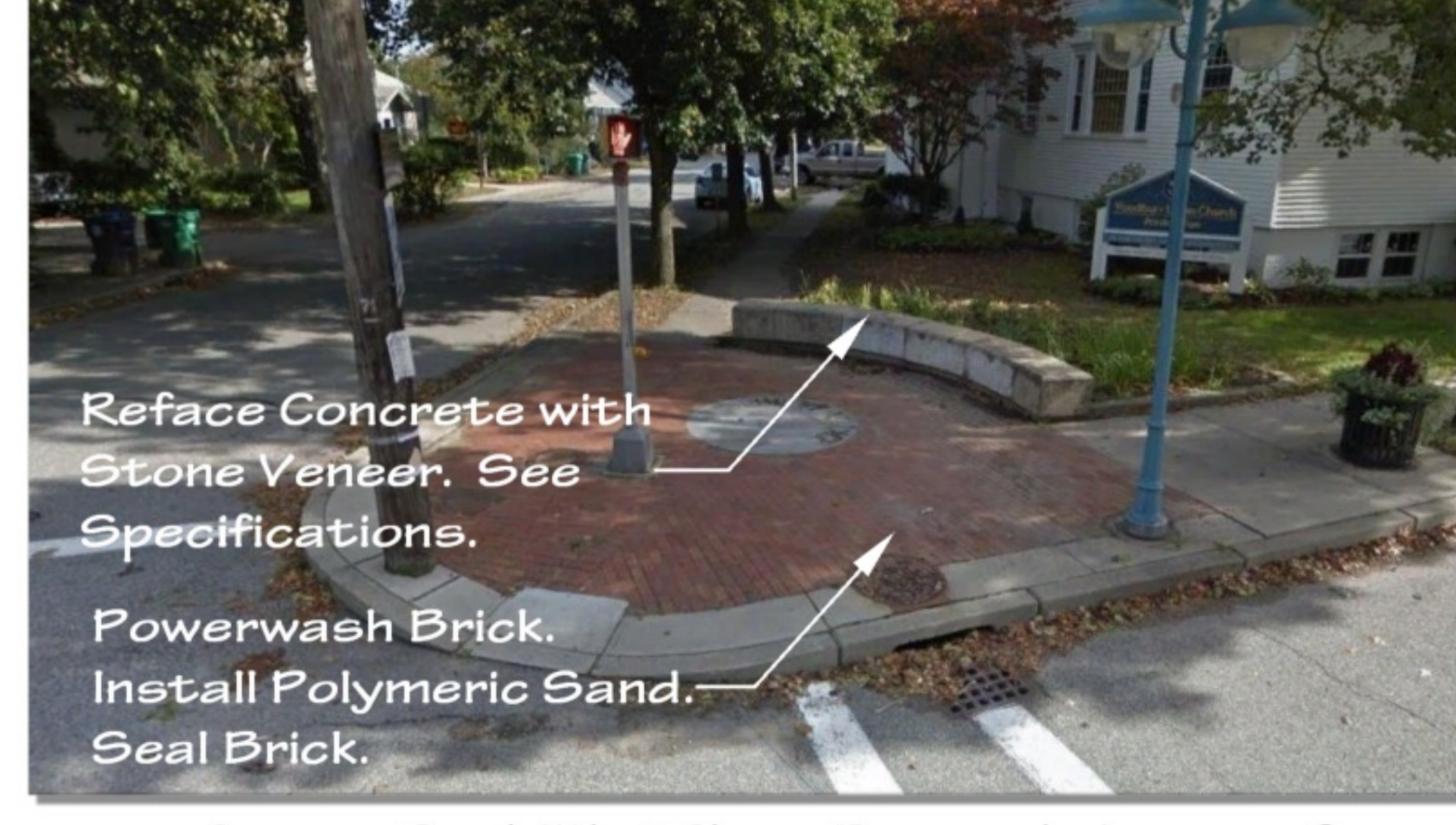
I Corner of Beach/ West Shore - Powerwash plaza area. Once dry install grey Alliance Super Sand polymeric sand or approved equal. Fill joints to flush with existing brick pavers in accordance with manufacturer installation instructions. Once dry, seal brick with Techniseal ProSeries Waterproofing Sealant for Brick and Concrete (WR7) or approved equal. Apply according to manufacturer recommendations.
