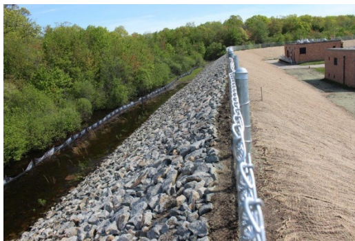
New levee to protect wastewater treatment plant from 500-year floods (2017).
