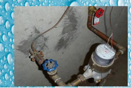
Identify the type of pipe coming into the building through the basement wall or floor as either plastic, copper,
